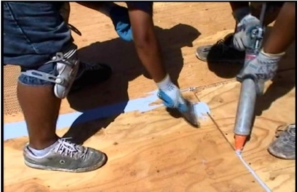
**#1** Caulk and Seal with E-101 Sealant all plywood joints. E-101 may be coated over immediately.
