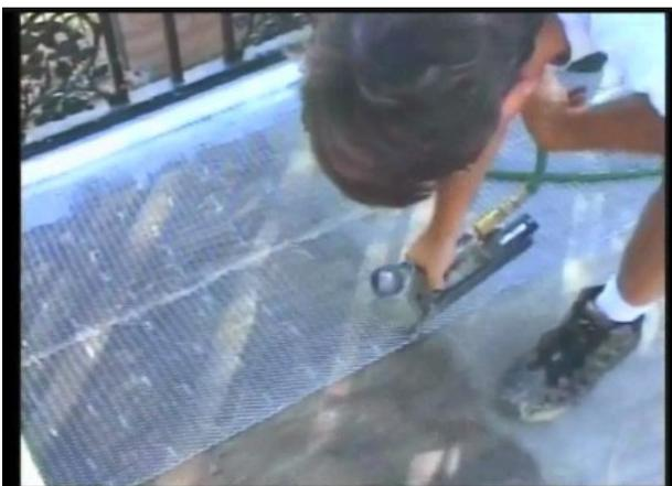
**#3** Staple down 2.5 lb galvanized diamond metal lath with 1" crown staples. Butt, do not lap metal lath. Make sure the lath lays flat against the deck with no void pocket voids under the lath. Overlap lath on flashing 1".
