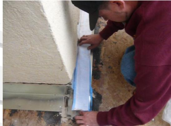
**#2** Apply Super Seal Tape to all metal flashings where coating is to be applied. The tape must be completely covered with coating.
